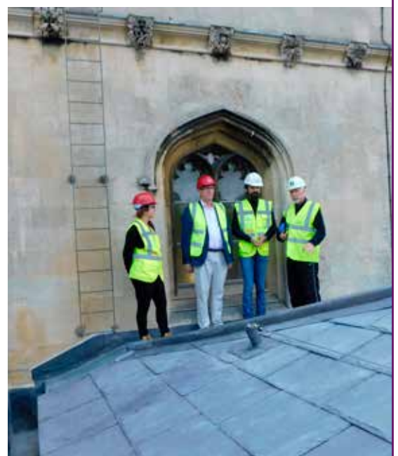
Provost Mike Proctor and Domus Bursar Phil Isaac inspecting the Library roof after completion
