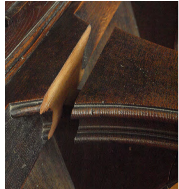
Split joinery - South Quire Stalls - High Stalls
