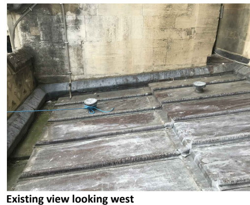
Existing view looking west
