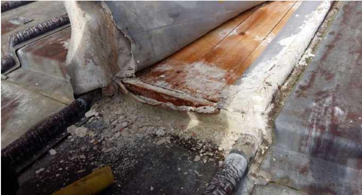
Opening up of the 1990 lead roof covering on Chapel N revealed substantial underside lead corrosion.
