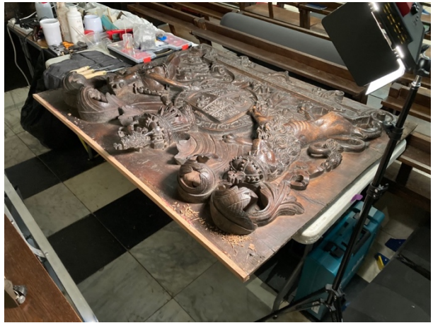
Elm fillet being fitted in position on top of the panel.
