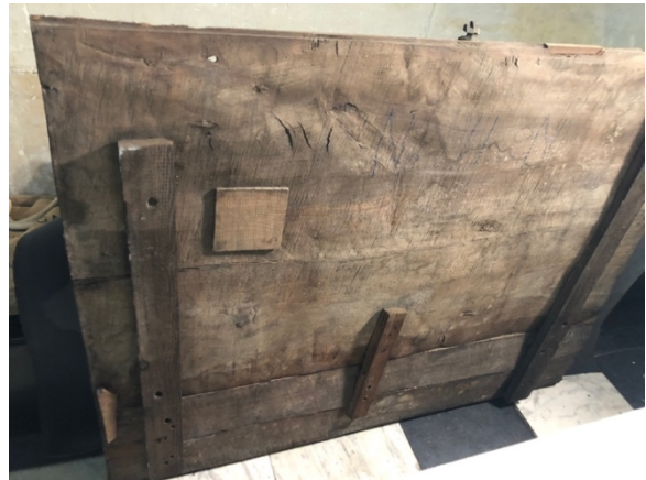
Back of the panel with various batten repairs
