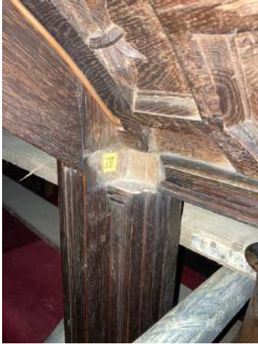
North, Chapel C bay B, loose moulding, low stall (before) And the same on North, Chapel C bay E low stall
