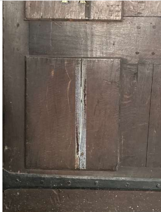
Bottom panel split – covered with gaffer tape residue
