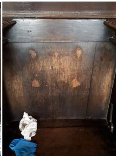
Damage on stall back, North Chapel C stall 2
