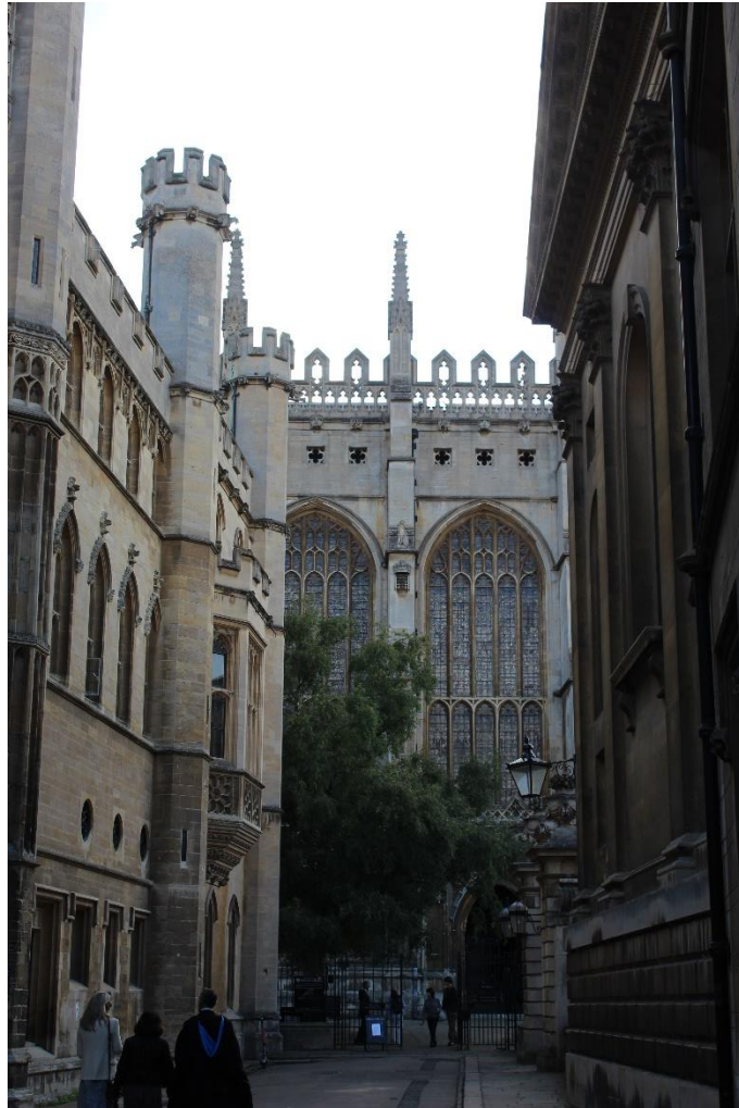
N façade, partial view from Trinity Lane
