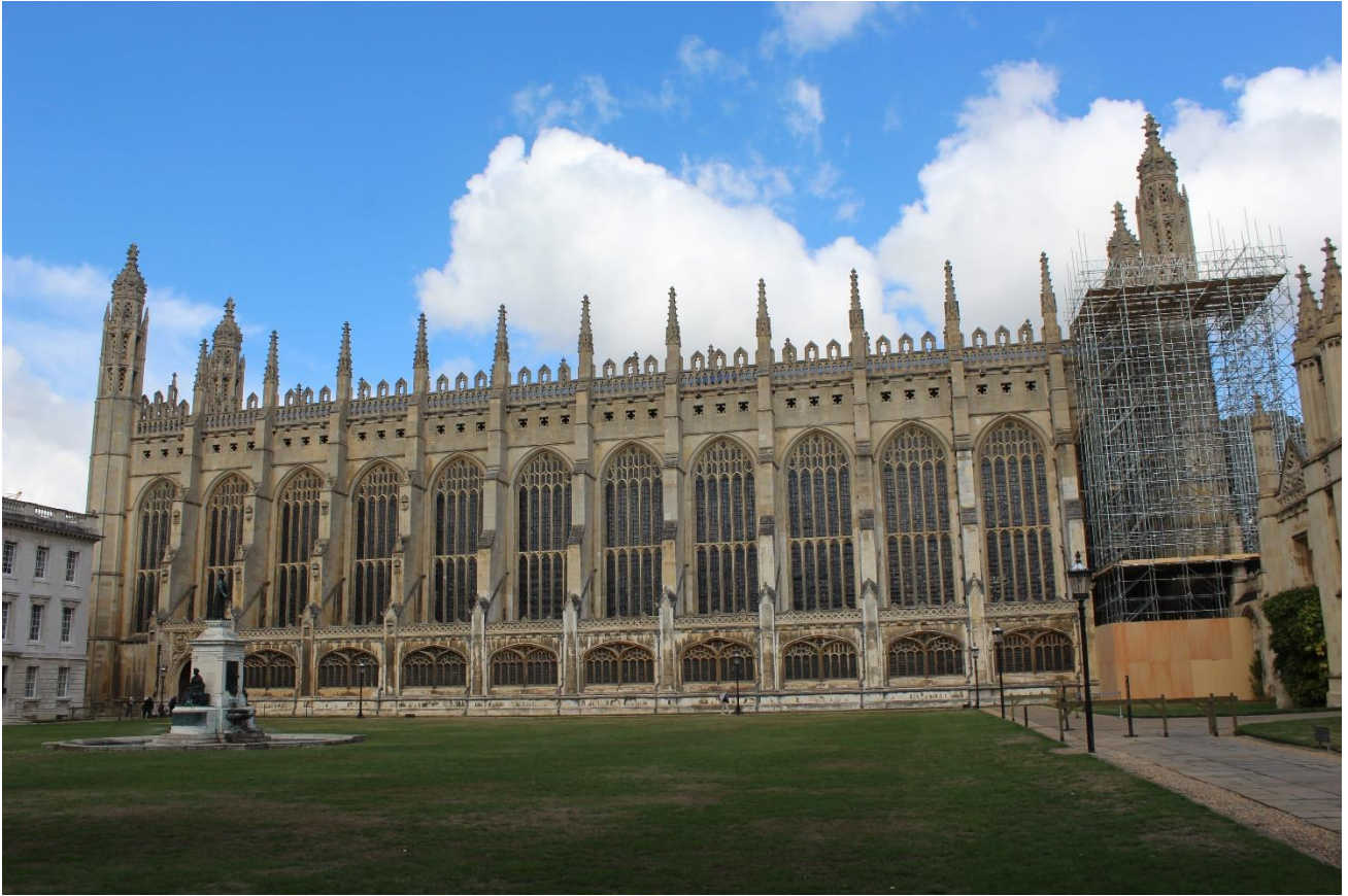
S façade from the far side of Great Court
