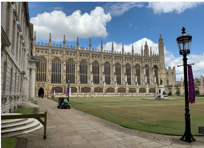
(Existing view before installation of the mock-up)
