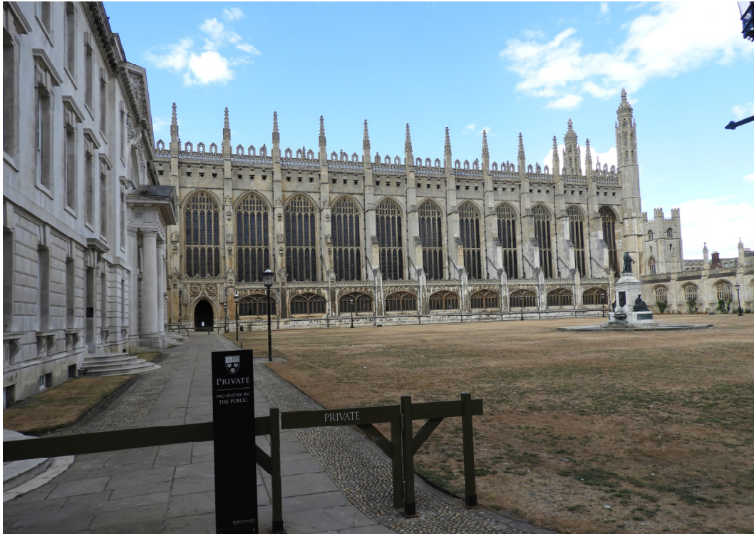
(Existing view with mock-up in modified position)
