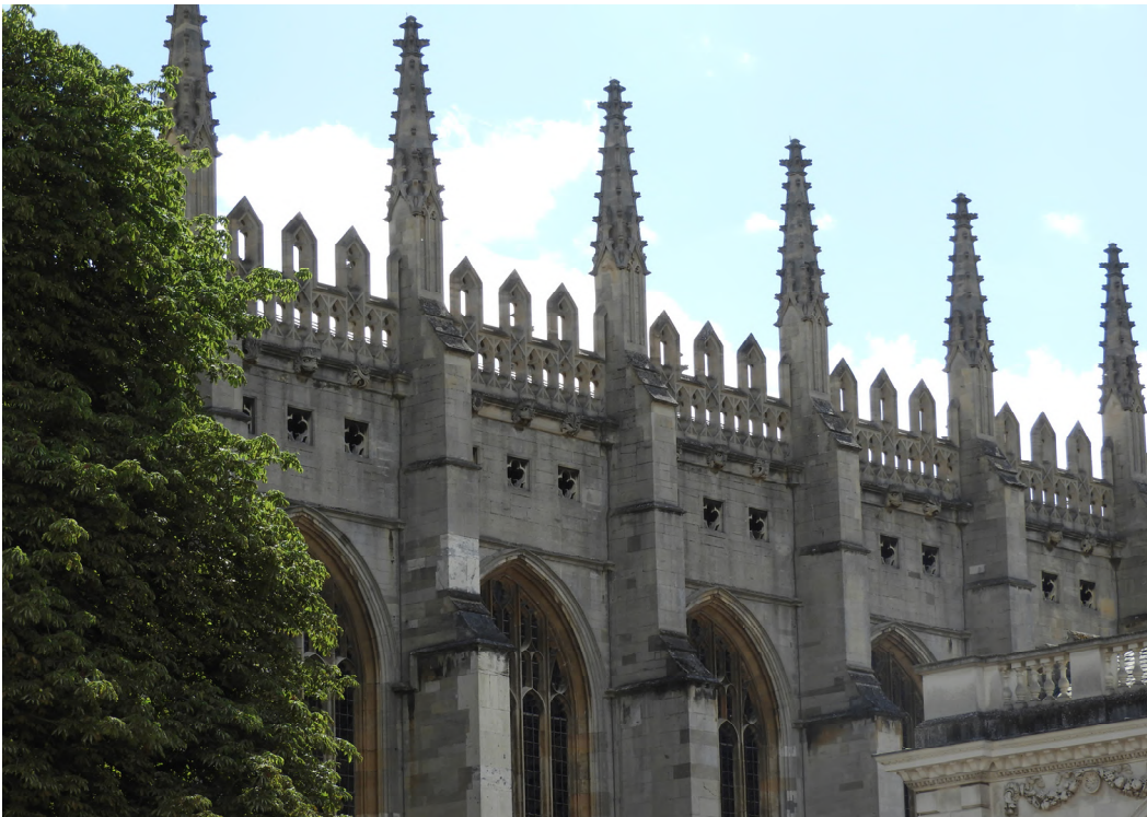
(Existing detail view)
