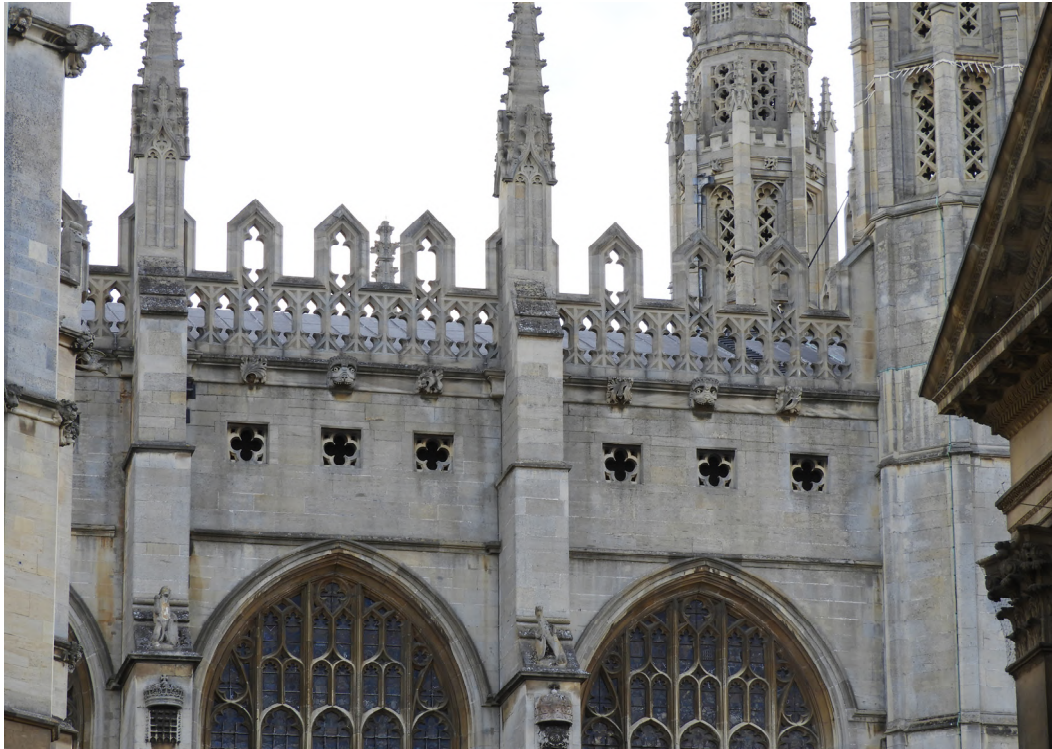
(Existing detail view)
