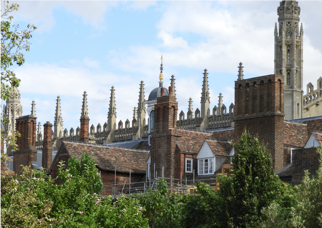
(Existing detail view)
