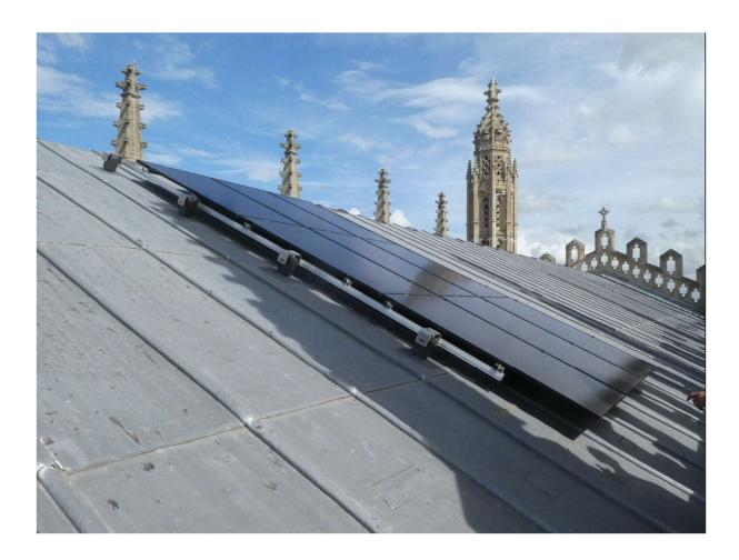
Views 2 and 3 – Views of the south slope mock-up taken within two minutes of each other. Note the darkness of the panels in the first image and their lightness in the second. (In both views there is also a shadow gap at the panels' foot.)
