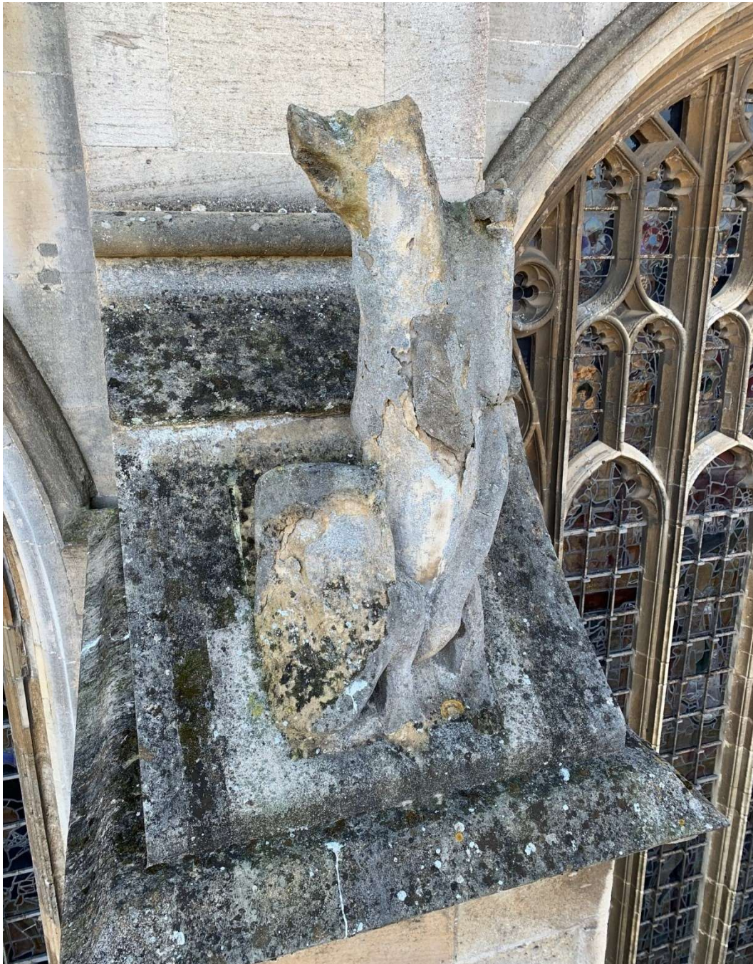
Loose and unstable carving on the buttress between bays 7 and 8.
