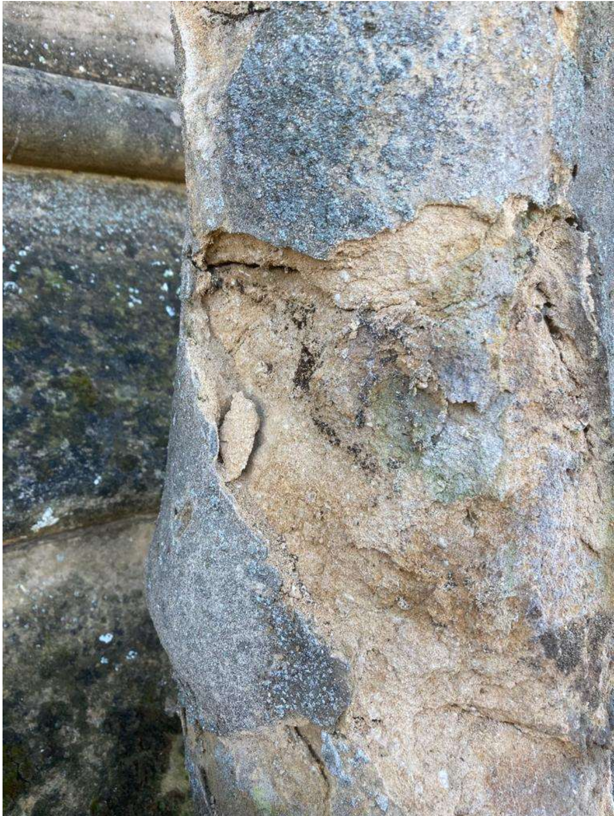
Detail of friable and cracked carving.
