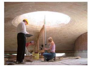
structural elegance and audacity of these wafer thin vaults, built without formwork or steel, captivated me - and I longed to build a tile vault in England. In 2003 I finally got the chance.
