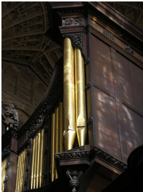
The collapsing front pipes before repair
