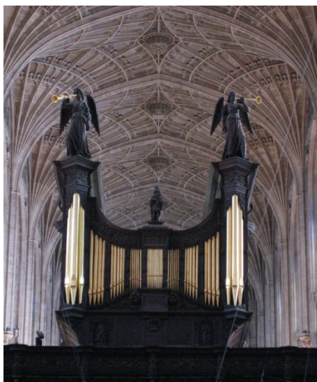
The west side of the organ case after repair of the south-west front pipes
